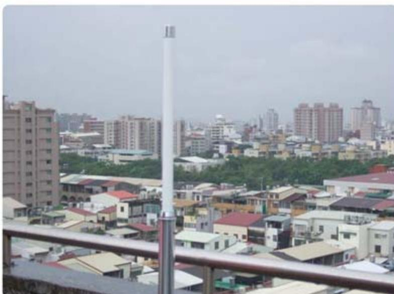
**Photo 3:** Take the antenna to the most remote end of the floor as to receive more WIFI signals.
